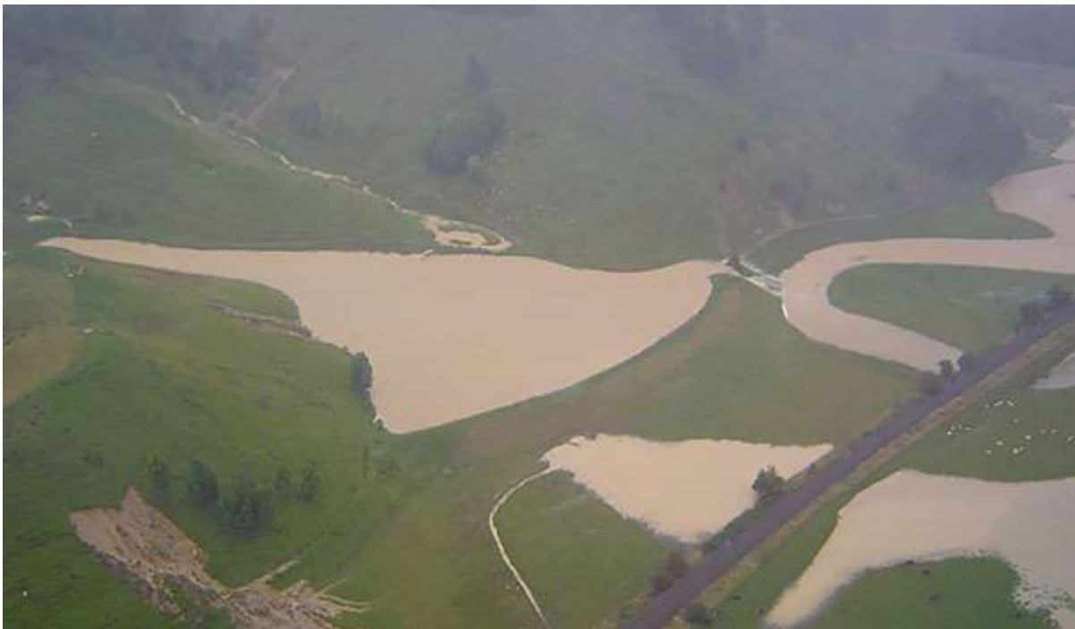
Photo: State Highway and North Island main trunk railway line near Hunterville protected by Porewa Dam during 2004 flood event.
