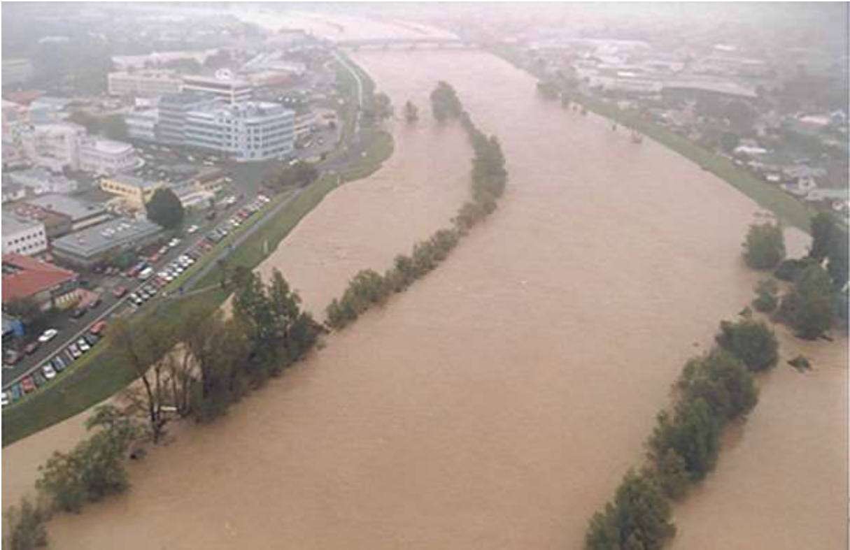
Hutt City centre with a 25-year flood event in January 2005
