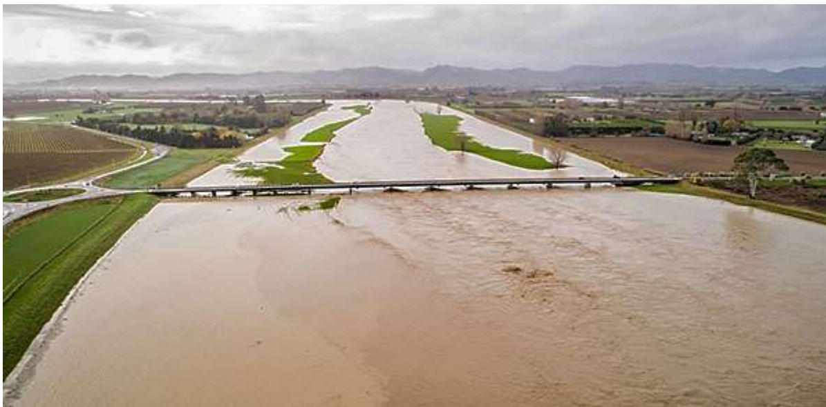
Waipaora River stop-banks containing 11 June 2018 flood event at State Highway bridge to Gisborne. NB Te Karaka township was cut off due to flood waters crossing the State Highway where there are no stop-banks.
