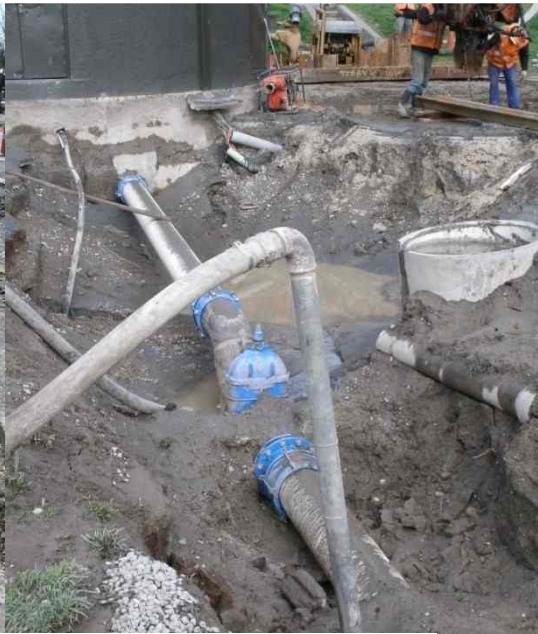
Replacing the rising main at Charles St
