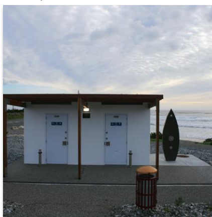
Public toilets supported by TIF
